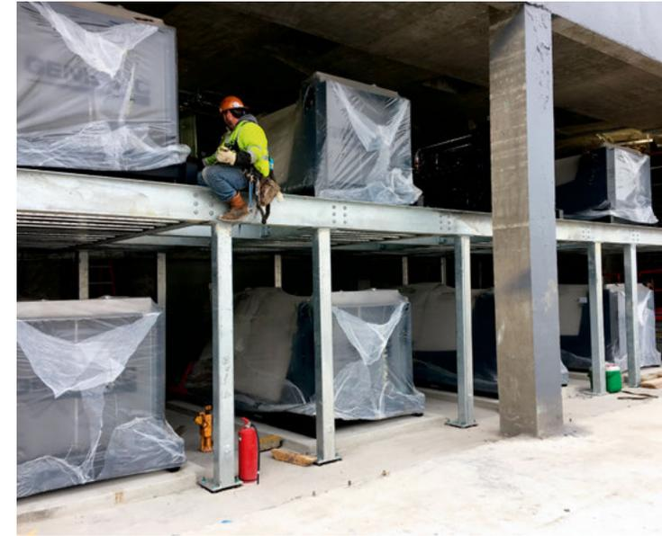
"This was a challenging application – a rooftop installation with natural gas fuel supporting life-safety and very important critical loads," adds John Sharpe, Power Solutions Manager for Generac. "We are pleased that the performance of the Generac natural gas generators and the design flexibility of our Modular Paralleling System could meet the project needs. Credit goes to the whole team for finding a creative and reliable generator solution for the owner."
